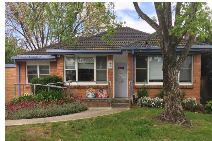
Kerrie Rd Neighbourhood House front entrance
